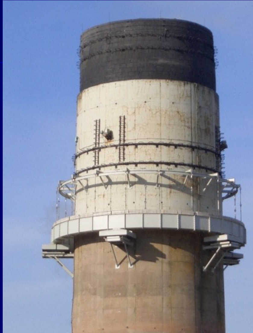
Fig 5 : TMD after installation
