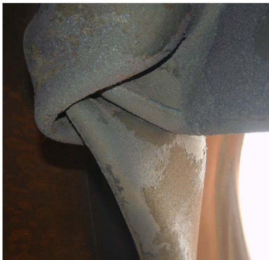
Photo 3 :detail of liner from inside.
