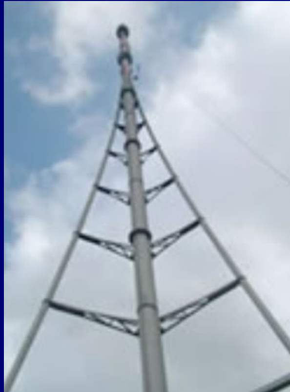
Figure 27 : very slender structure (136 m) requiring a damper system for the second vibration mode.
