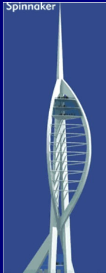
Figure 29 : Spinnaker 170 m high rise building
