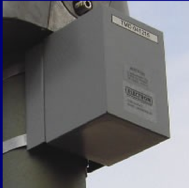
Figure 41 : detail of a light pole damper
