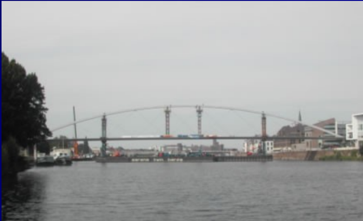
Figure 36 : very slender bridge supposed to vibrate vertically as a result of pedestrians walking on it.
