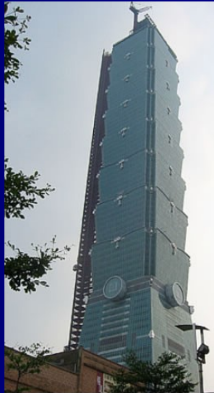
Taipei 101 under construction, July 2003
