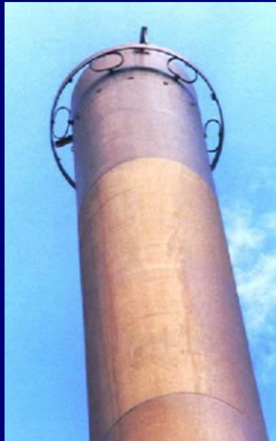
Figure 13 : stack with a TMD - damping elements made of cables
