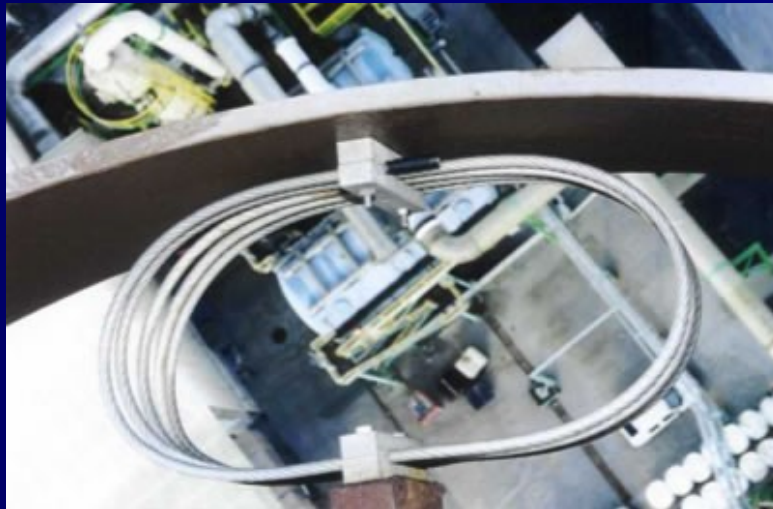
Figure 14 : detail of the cable-damping element
